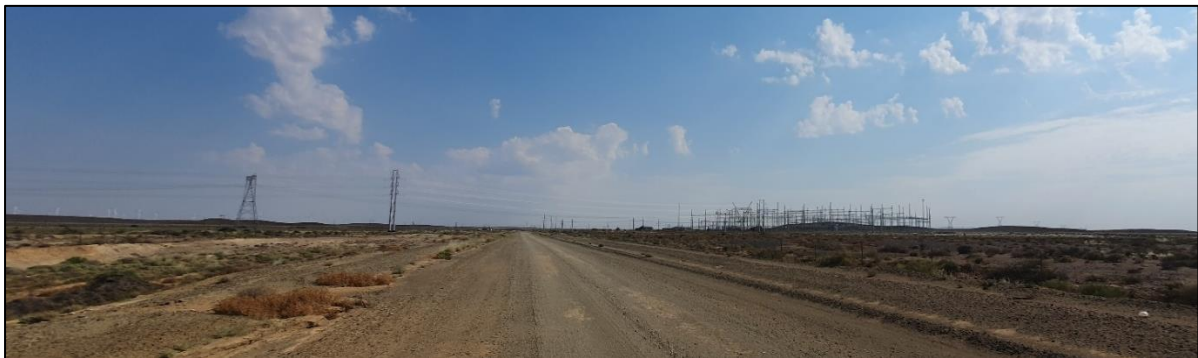
Figure 44: Existing network of powerlines converging at Helios MTS
