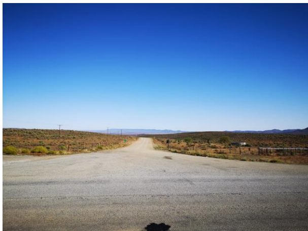
Image 5-1 R355 at intersection with R357
