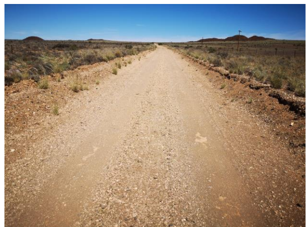
Image 5-12 Typical condition of PR1
