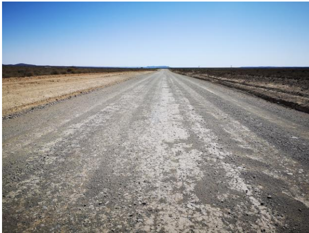
Image 5-5 Typical condition of AP2972
