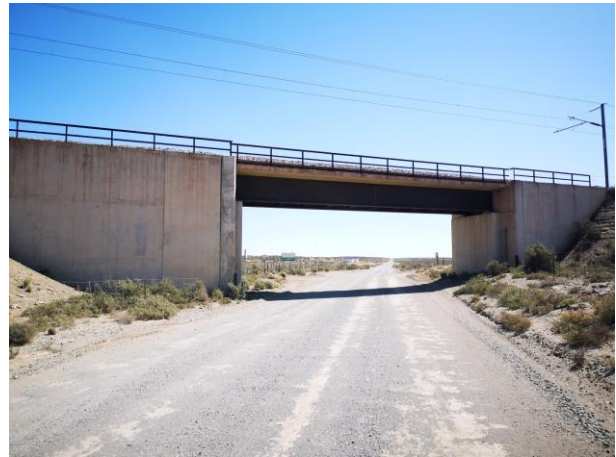
Image 5-6 Railway bridge over AP2972 before TR1
