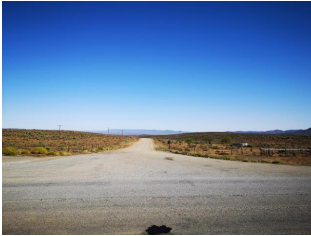
Image 5-1 R355 at intersection with R357
