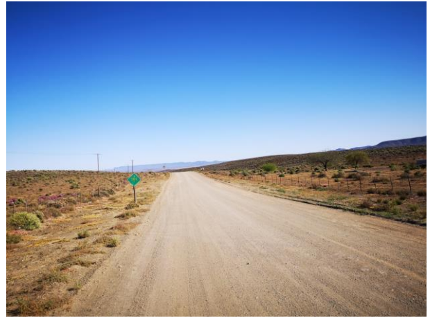
Image 5-2 Typical condition of R355
