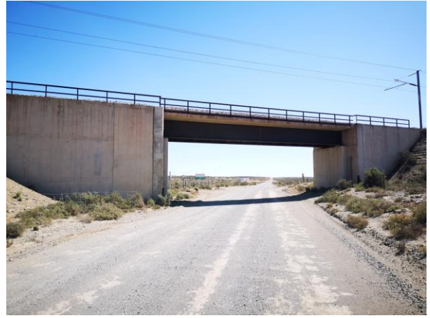
Image 5-6 Railway bridge over AP2972 before TR1
