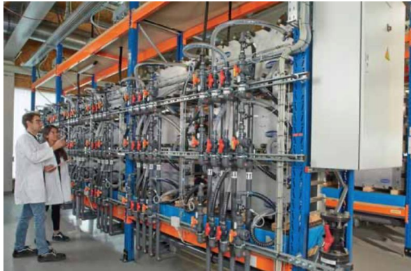
Stacks of a 2MW/20MWh vanadium redox flow battery at Fraunhofer ICT. Image:
