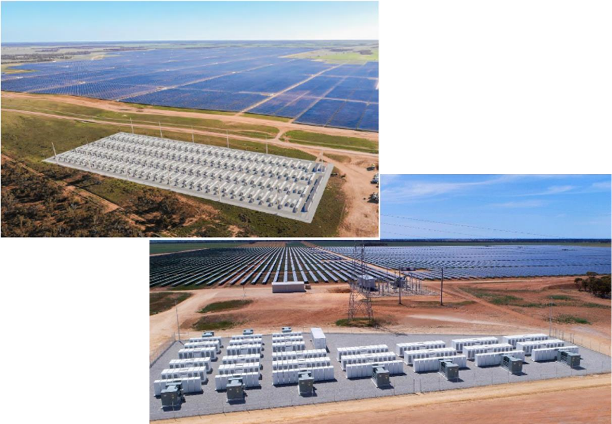
FIGURE 2.3.1.1 – Images of Typical BESS Systems Servicing Solar Power Farms
