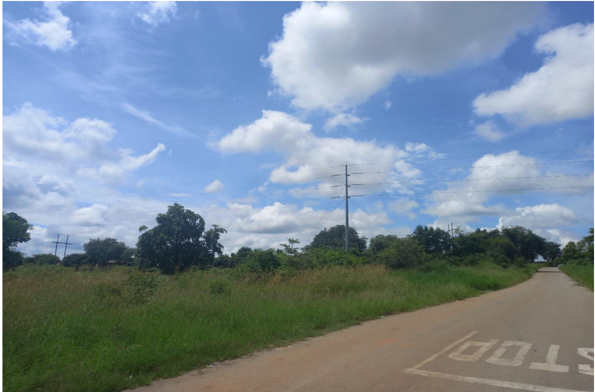
Figure 6: View of some of the roads that will be crossed by the powerline.
