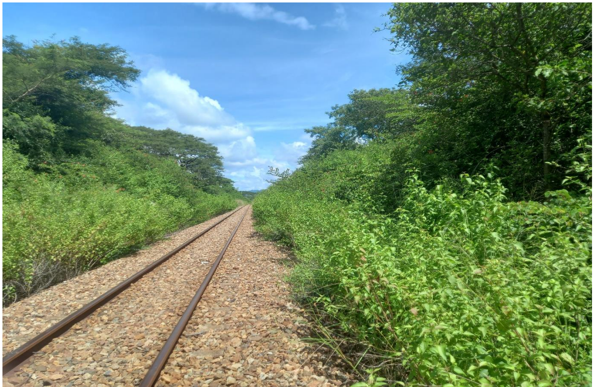
Figure 5: View of the railway line: the new line will run parallel to it for most of the part.
