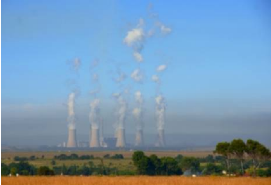
Figure 4.5: View of Lethabo Power Station from the agricultural areas to the south east.
