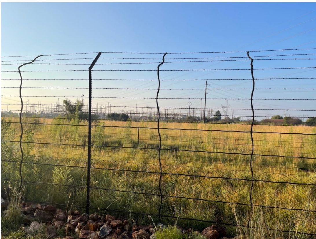
Figure 5. Eskom Watershed Substation.
