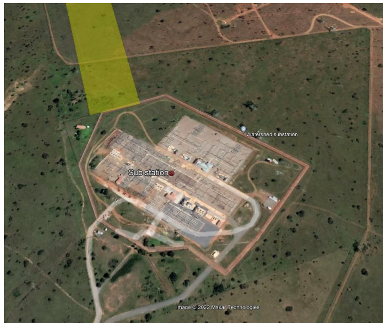
Figure 2 Watershed Power Substation
