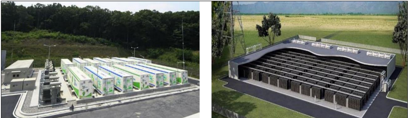
Figure 6. Battery Energy Storage System (BESS)
