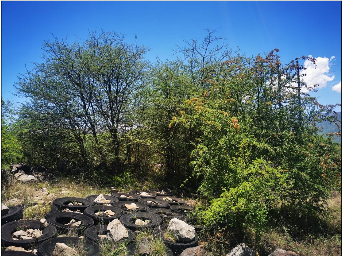
Figure 33: Illustration of tyres used for erosion control
