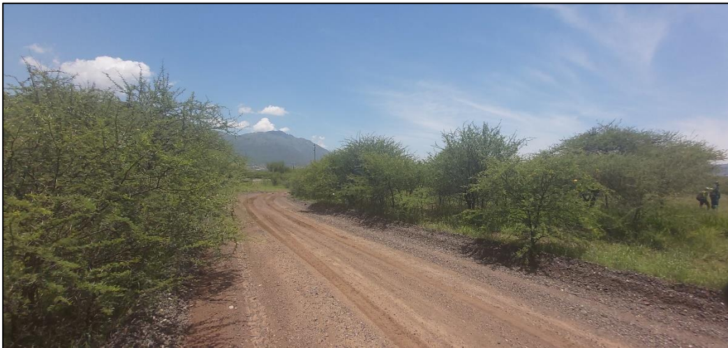
Existing access roads towards the R 555 (looking southwest from the site).
