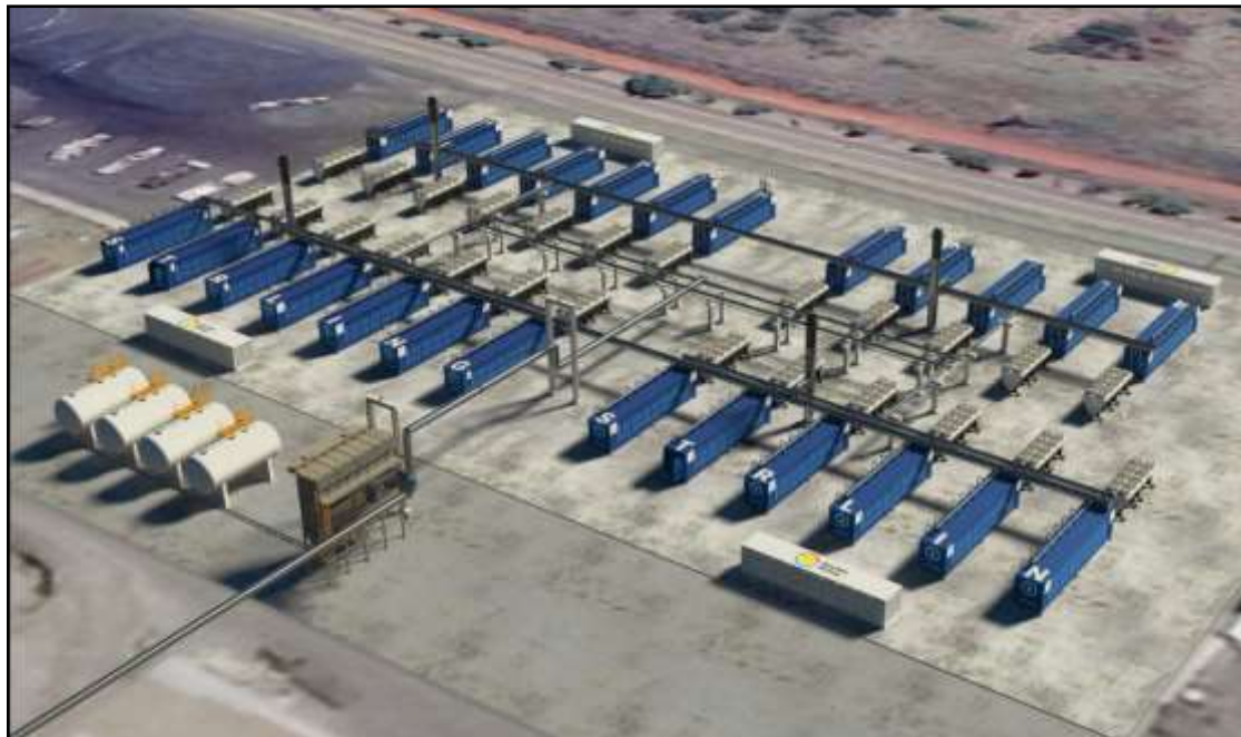
Figure 5: Aerial view of an ECF.
