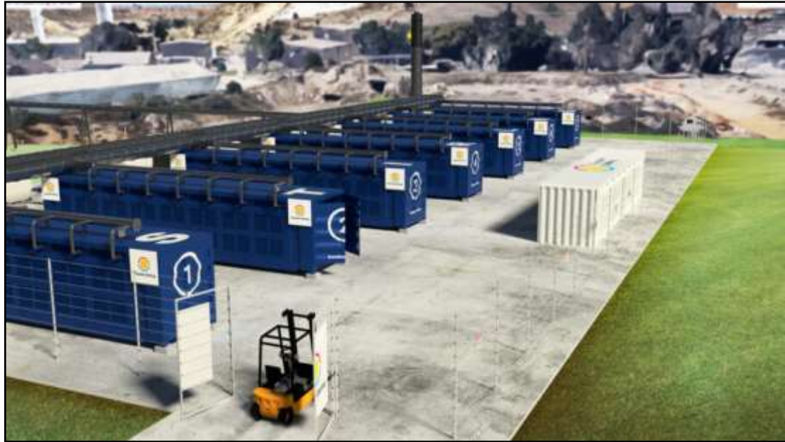
Figure 4: Close up view of an ECF.
