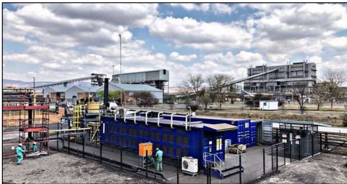
Figure 3: Construction of an ECF.
