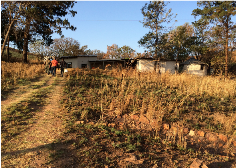
Hondekraal gate picket to be demolished
