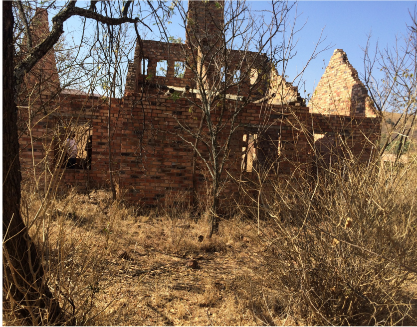
Hondekraal valley existing structures to be finished
