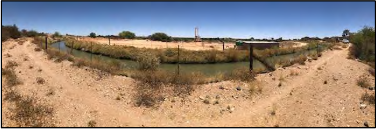
Canal at the point where the proposed new balancing dam will be constructed.
