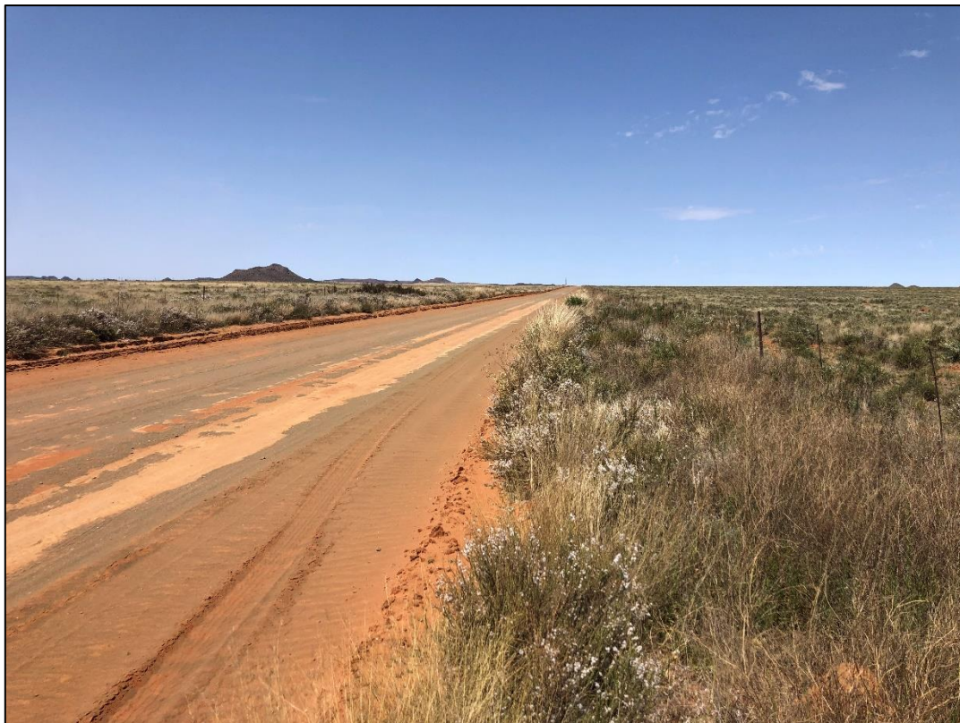
Plate 9: Access roads SE towards town of Luckhoff
