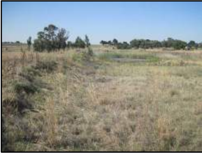
Figure 5. General Site conditions – Earthen dam
