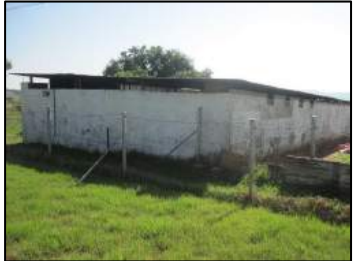
Figure 6. General site conditions. – Existing piggery
