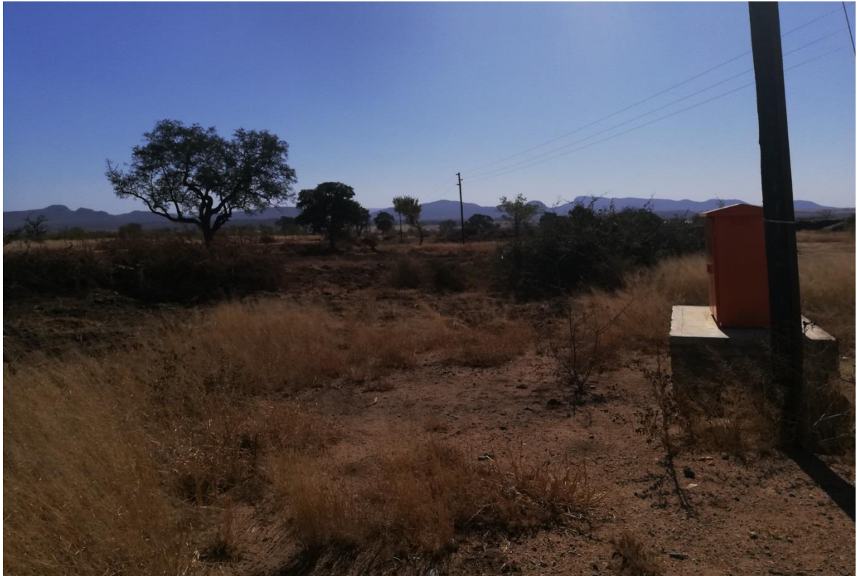
Existing powerline and vegetation around the farm
