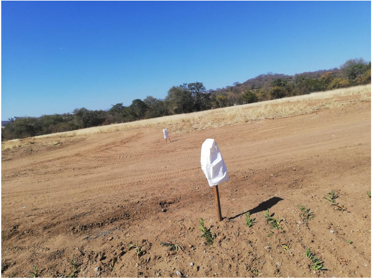
Picture showing the pegs where the poles will be planted
