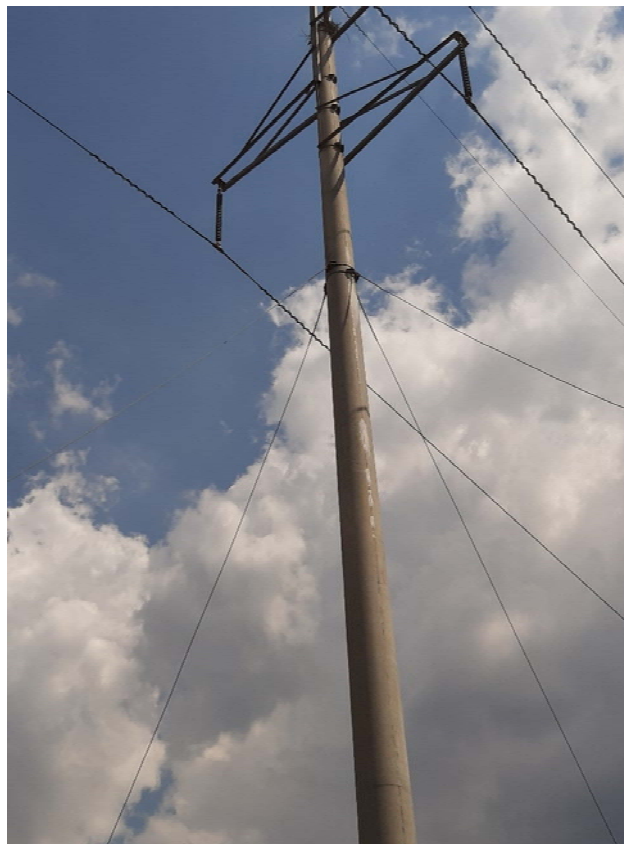
Figure 8: Example of a steel monopole structure noted on site
