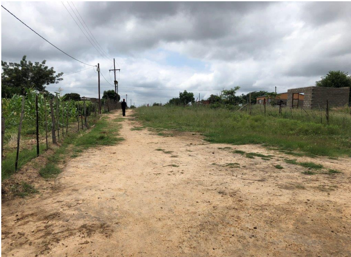
Picture 4: Shows the existing powerlines in the area
