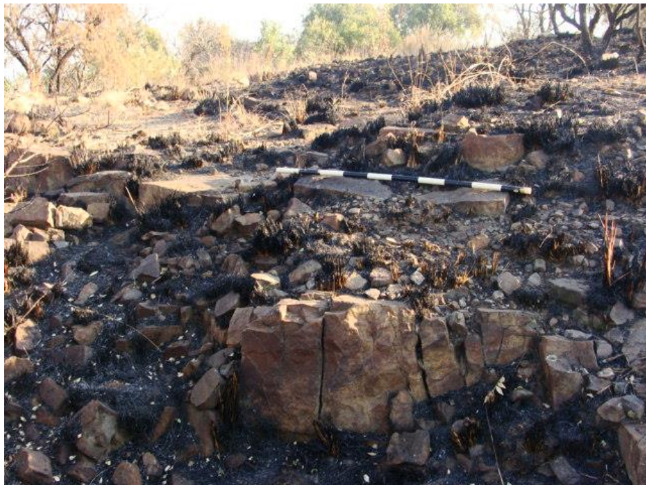
Figure 6 Corner junction between wall on the western and one on the southern side.
