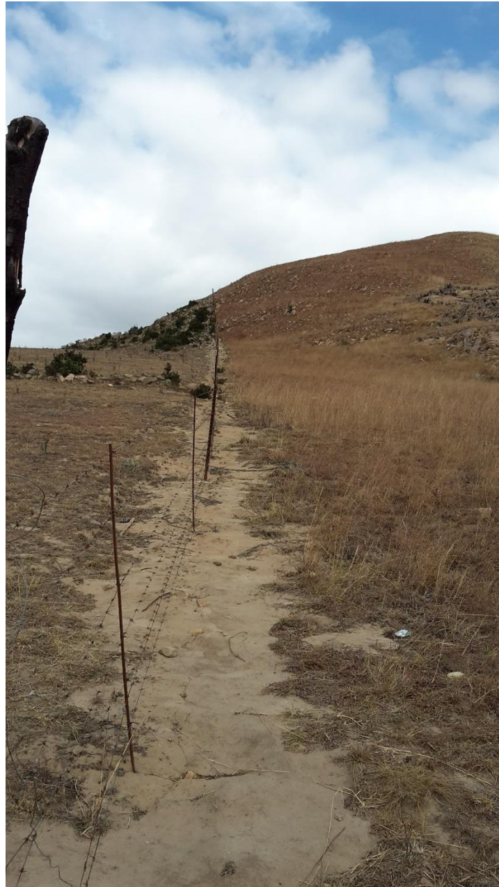
Figure 11: Border fence condition from Oshoek to the Komati River
