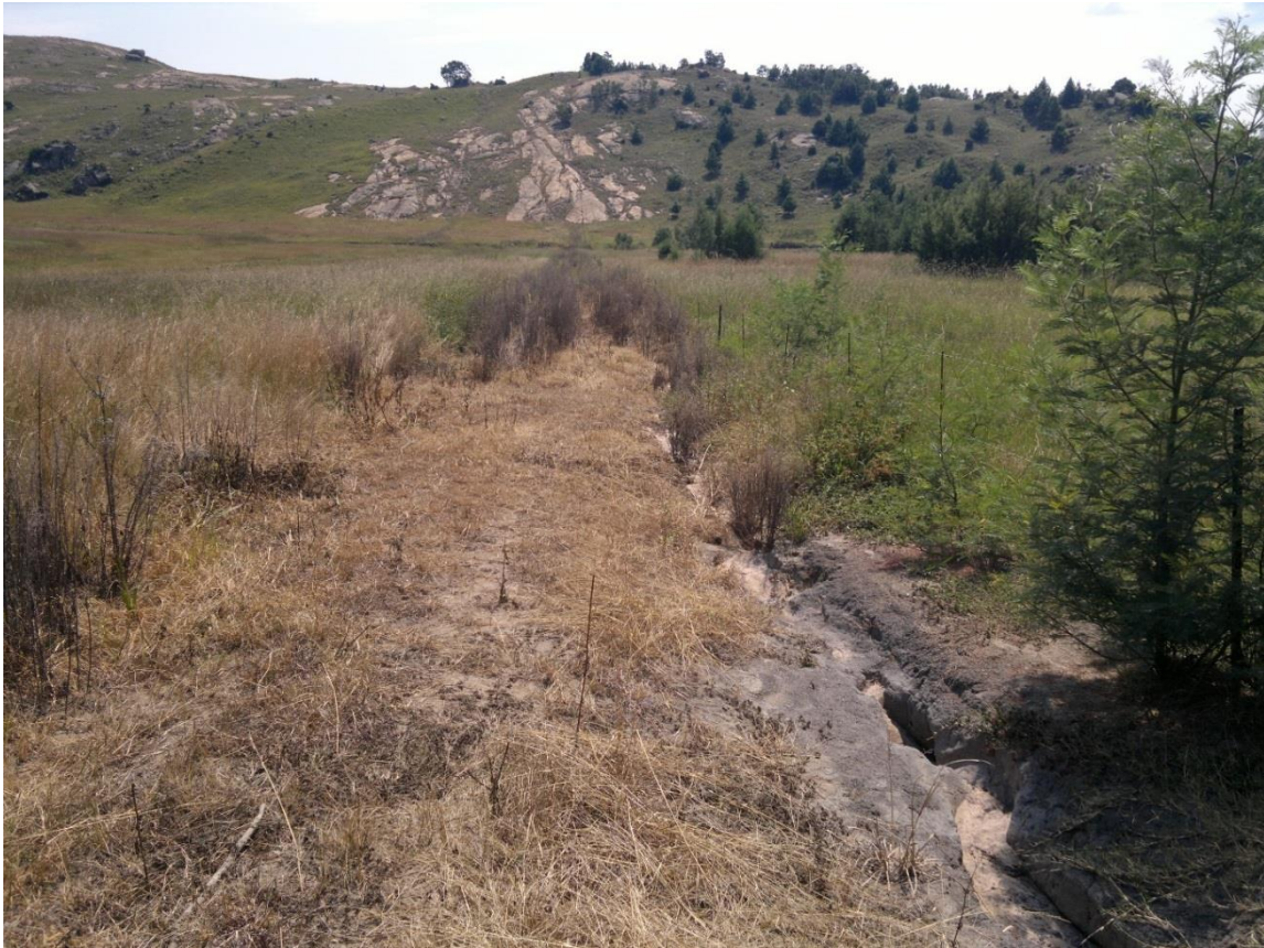
Figure 10: International border fence and disused track in the area north of Nerston
