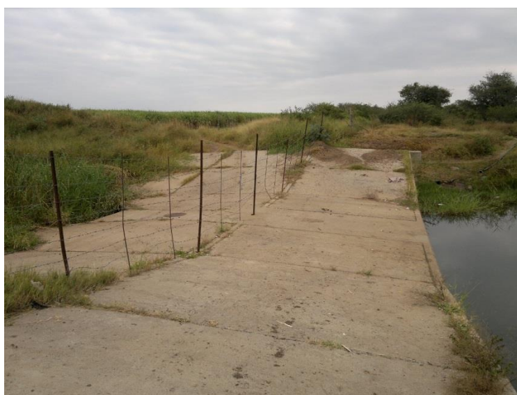
Figure 13: Old culvert structure and international fence in the Mananga area
