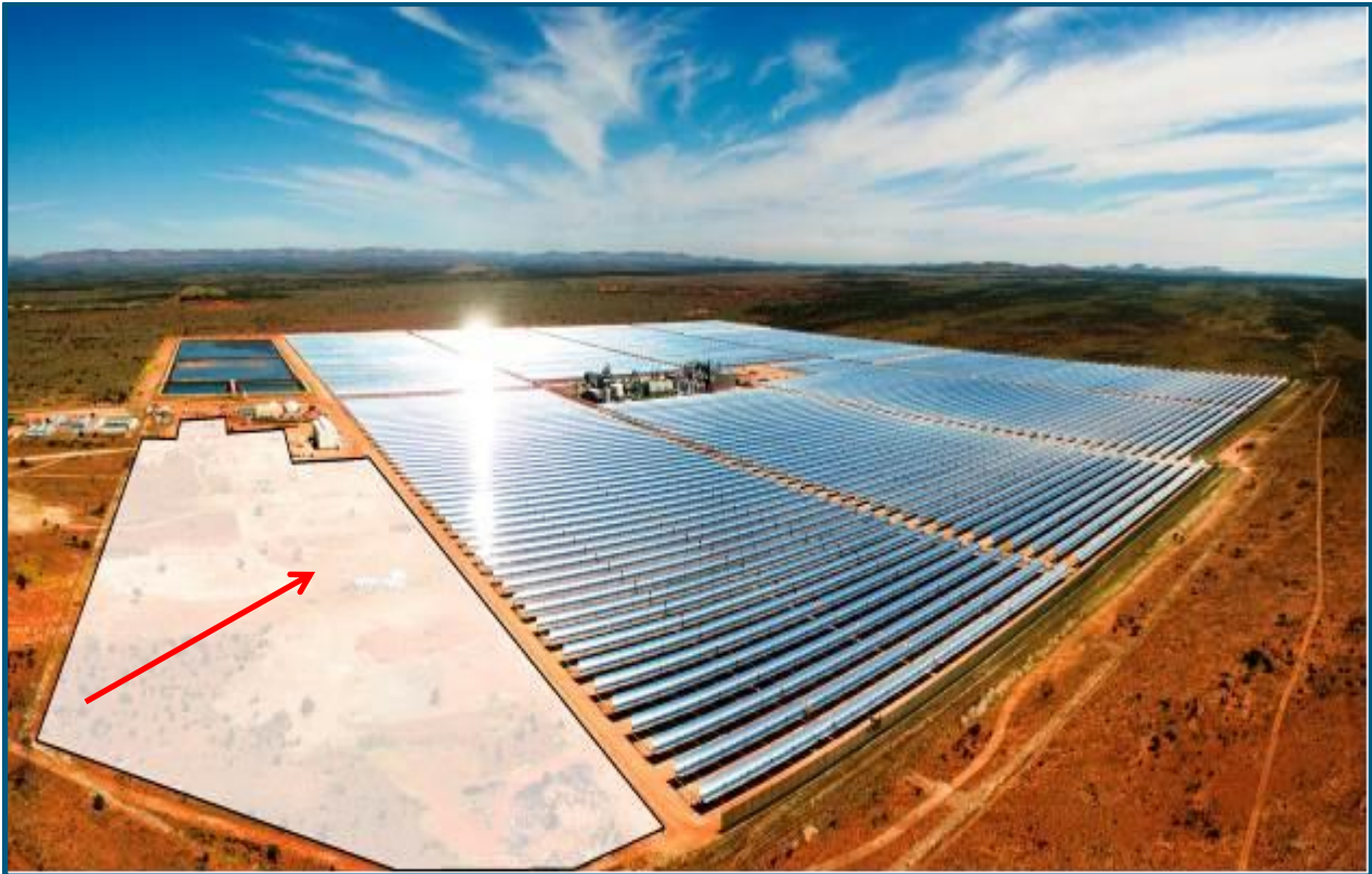
Figure 3: Location of the 4MW Power Plant
