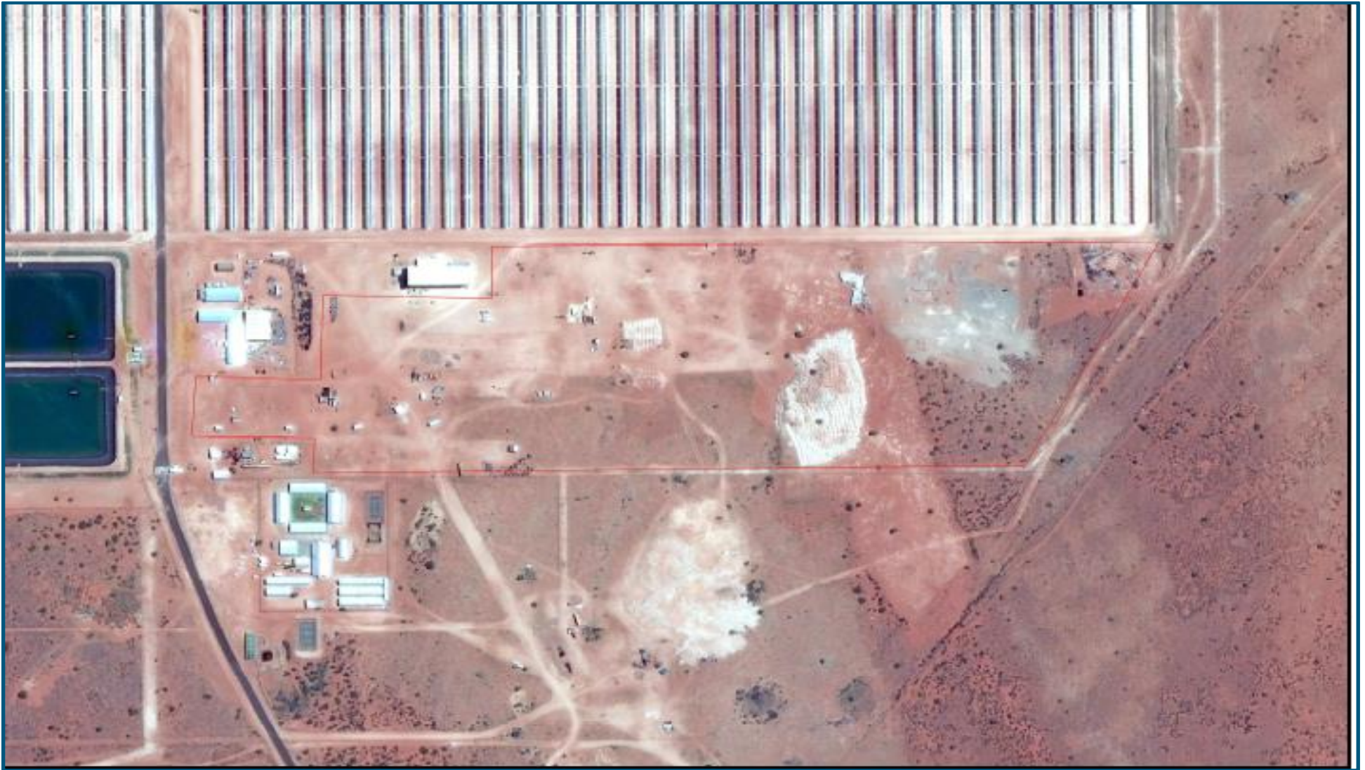
Figure 9: Status of the Footprint for the 4MW PV Plant
