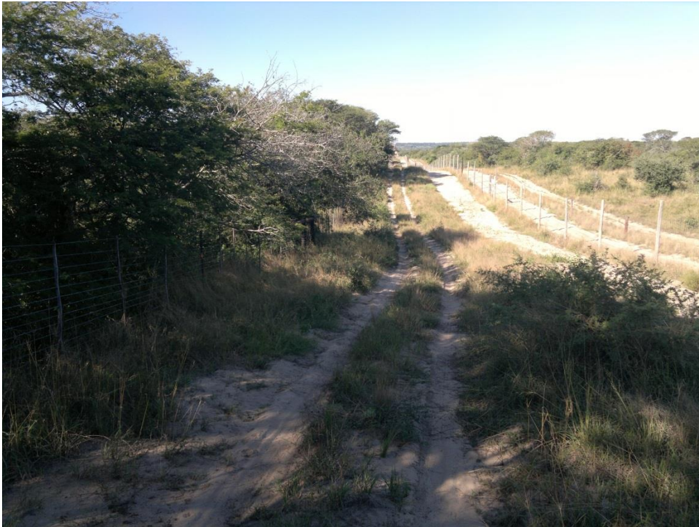
Figure 3-8: Existing international border fence (far left) and patrol track (centre), with the Tembe Elephant Park boundary fence, inner electric fence and patrol tracks (right) in the Tembe Elephant Park
