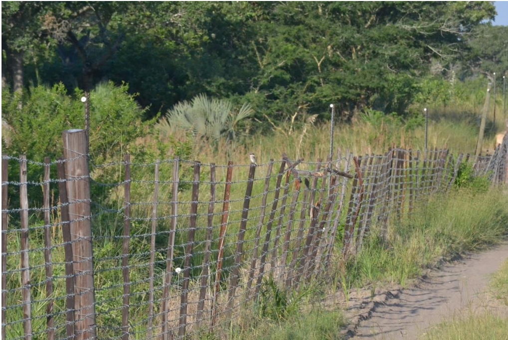
Figure 3-6: Existing fence damaged by elephants east of the Tembe Elephant Park
