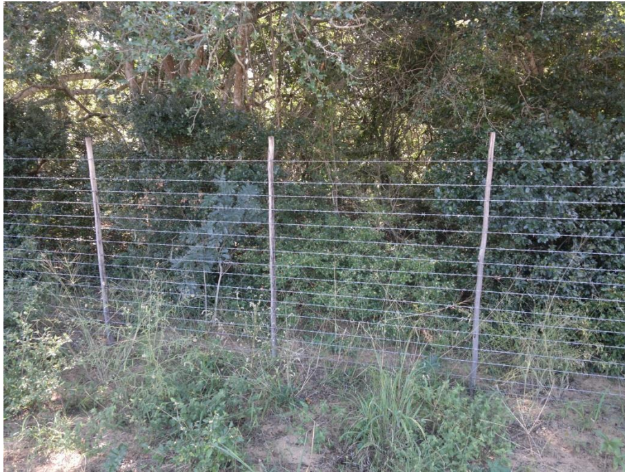
Figure 3-2: Example of the existing fence along the Mozambique-South African border in the Tembe Elephant Park
