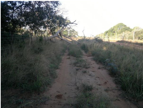
Figure 3-5: Existing fence in states of disrepair – damaged by a fallen tree in the Tembe area (left) and the damaged by people crossing into Mozambique east of Tembe (right)
