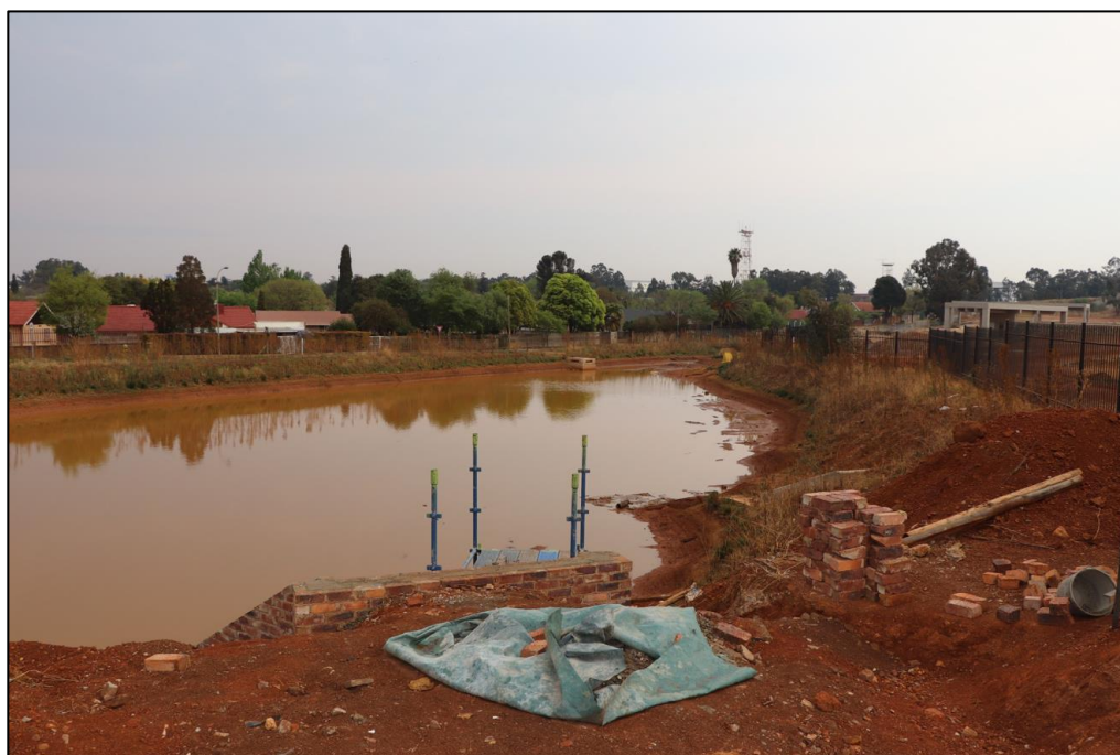
Figure 5-2: Attenuation pond/ dam located in south-eastern corner of existing JMP site
