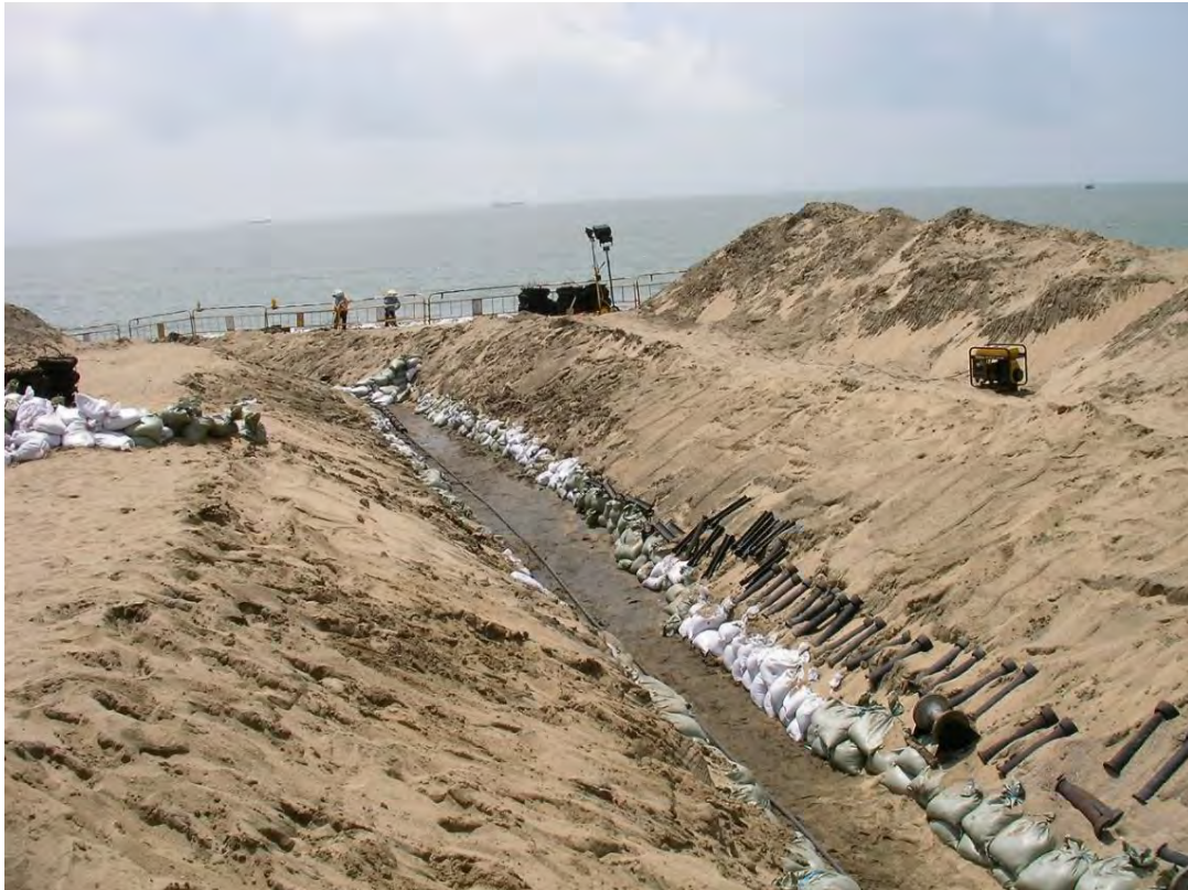
Figure 2-25 Example of Subsea Cable Installation by Trenching
