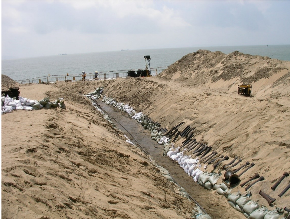
Figure 2-18 Example of Subsea Cable Installation by Trenching
