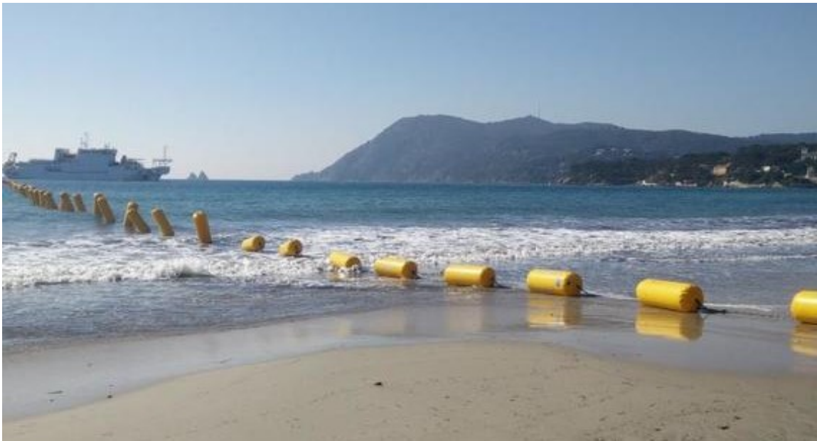
Figure 2-15 Example of Installation of the Subsea Cable in the Nearshore
