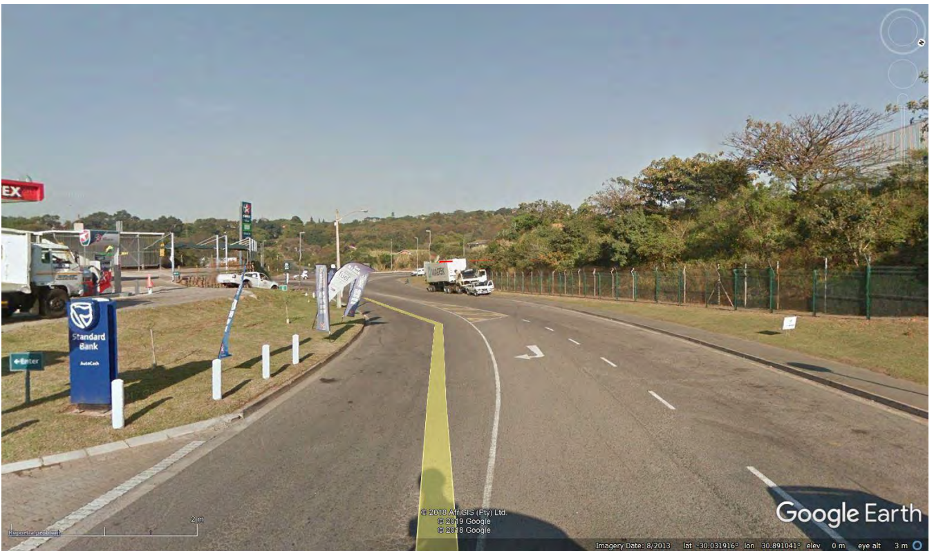
Plate 10: Options 1 & 2 - view south along Ashgate Road from entrance road to Southgate Industrial Park
