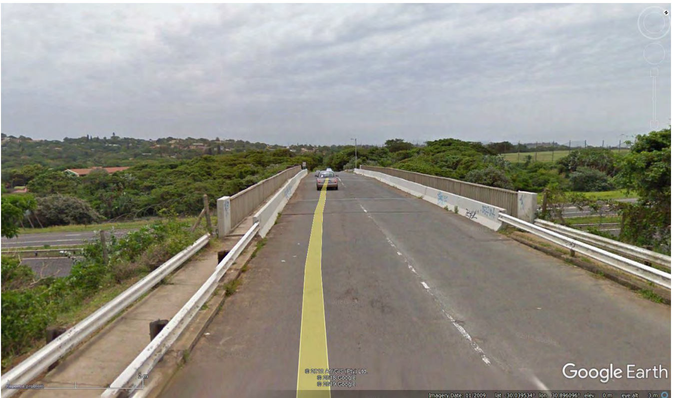
Plate 6: Options 1 & 2 - view north-west across Umdoni Road bridge over N2
