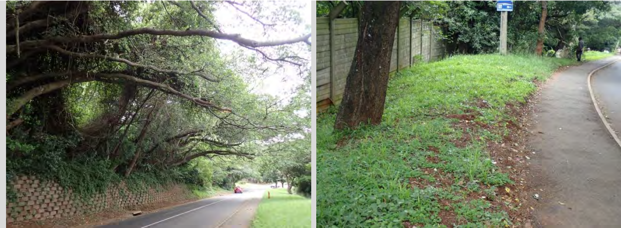
TCR 2 (Segment H) - 30.034655°S, 30.888664°E to 30.033090°S, 30.889873°E
