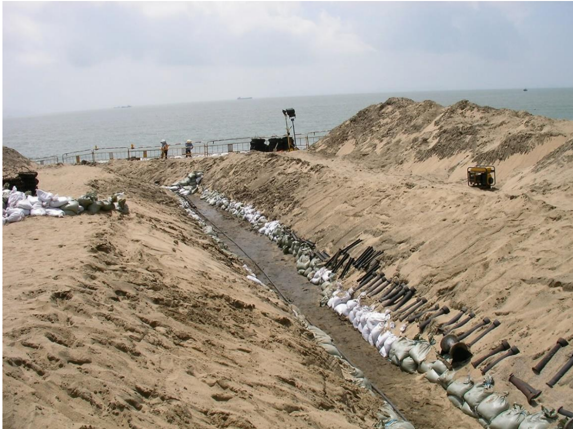
Figure 2-24 Example of Subsea Cable Installation by Trenching
