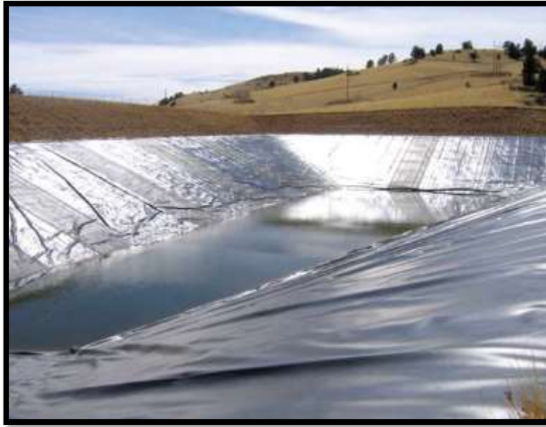
Figure 28: Lined pollution control dam (PCD) illustration
