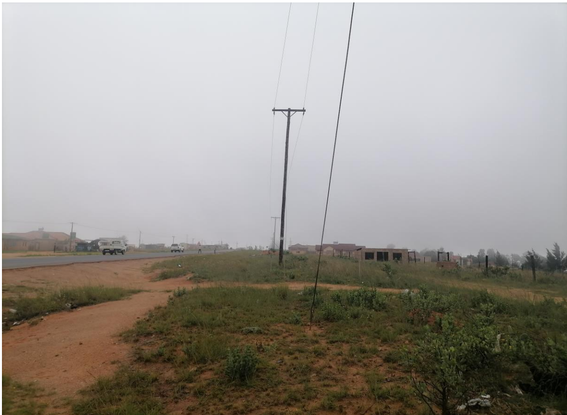
Photo 4: Existing powerline where the new powerline will T-off
