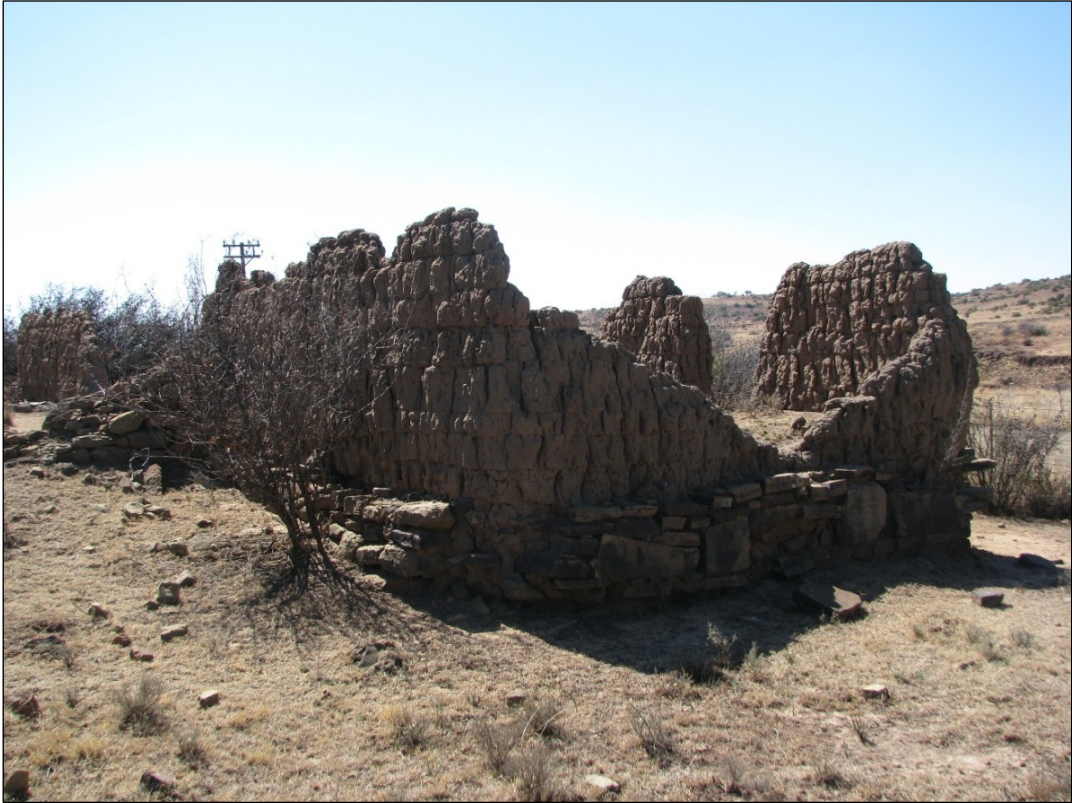
Figure 7: The remains of the main structure (house) at the site.
