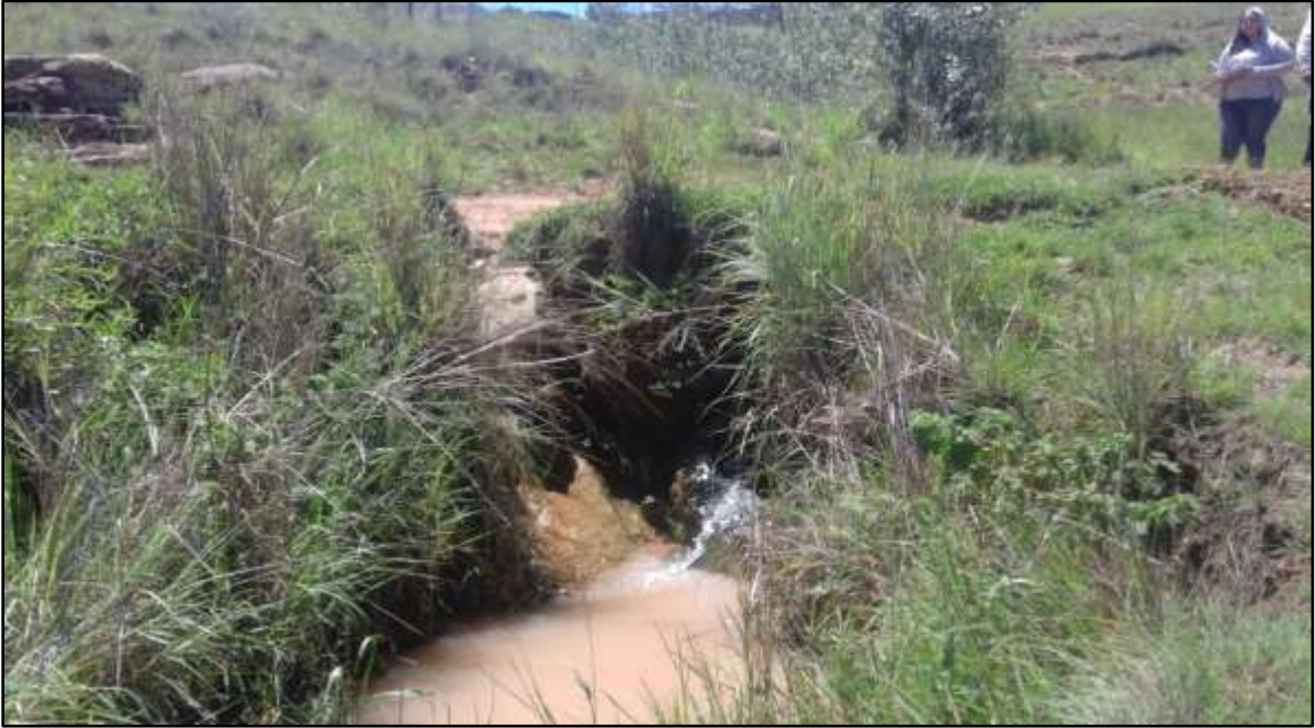
Photo 1: Showing the existing structure at Watercourse No.01
