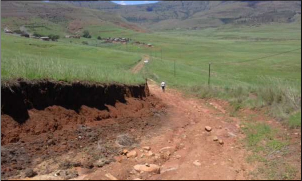
Photo 3: Showing the undercutting of slopes and the erosion along the existing route.
