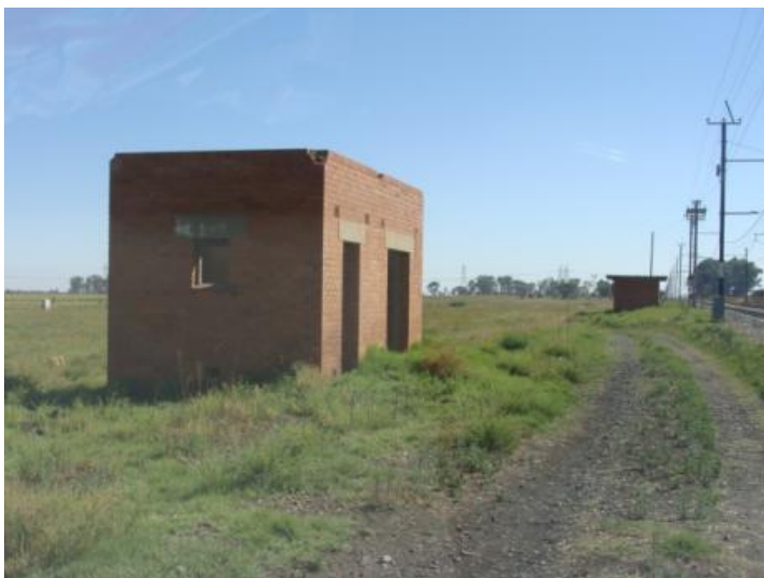
Figure 4.7: Station buildings at site no. 2
