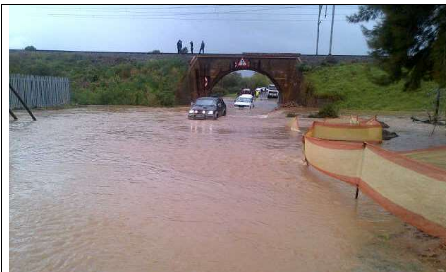
Figure 7: Flooding of the Van Wyks River under the railway bridge at km 0,2 (August 2013).
