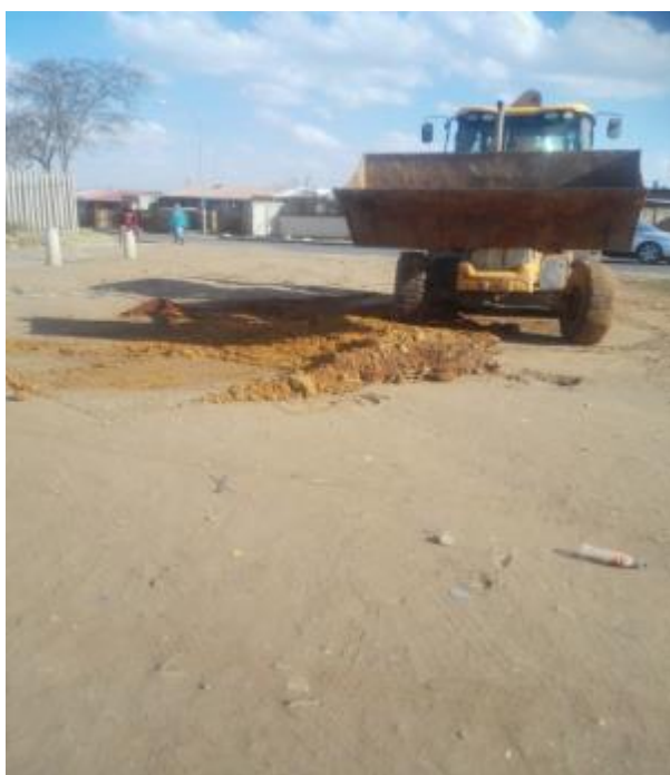
PIC A: The TLB used to excavate test pits
