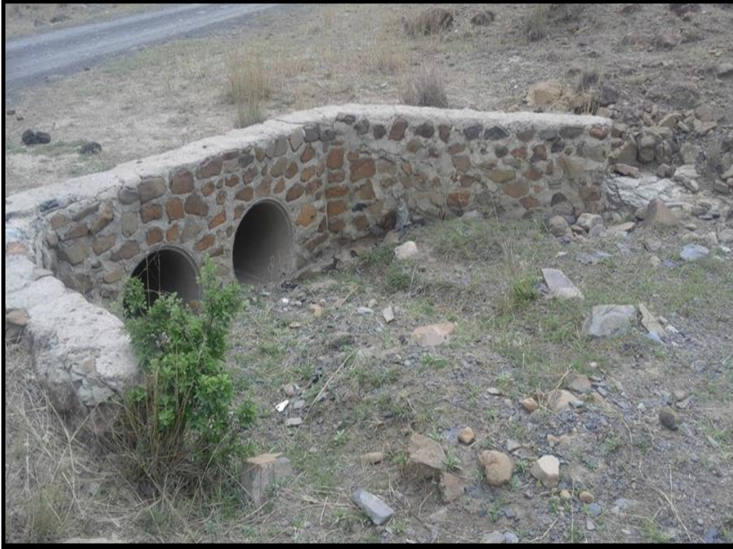
Photo 3: Showing stone pitched pipe culverts with headwalls
