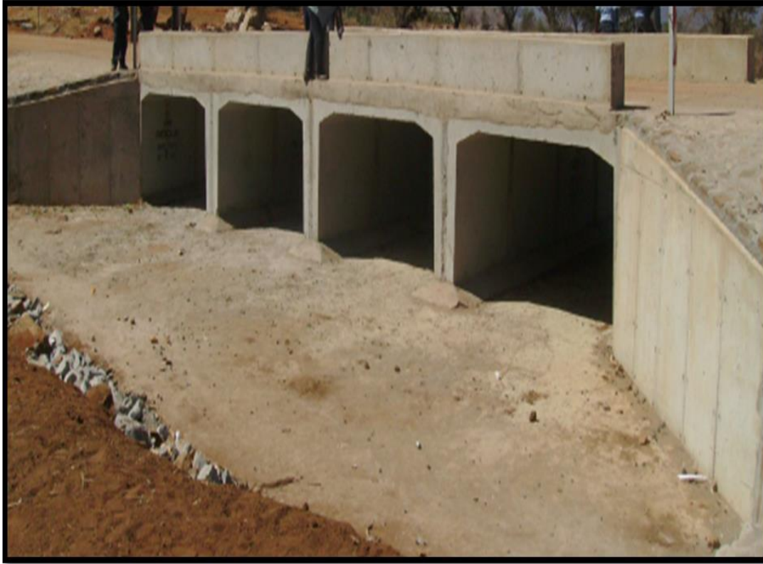
Photo 2: Showing an example of a portal culvert causeway structure
