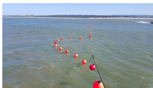
Plate 10 Bringing the cable to shore from the cable laying vessel. Cable is buoyed off and pulled to shore with smaller vessels.
