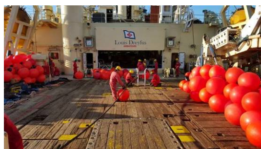
Plate 10 Bringing the cable to shore from the cable laying vessel. Cable is buoyed off and pulled to shore with smaller vessels.
