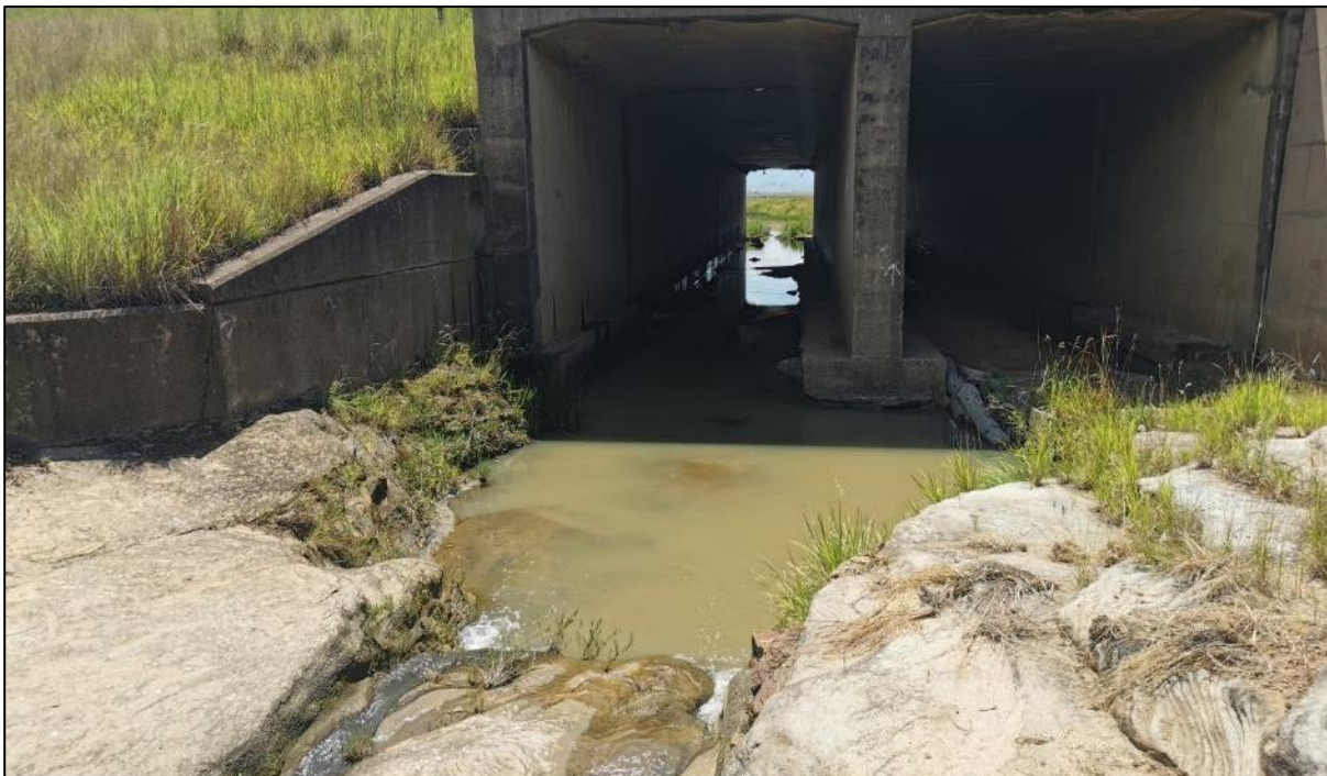
Figure 44. A structure within a watercourse in the study area (February 2022).
