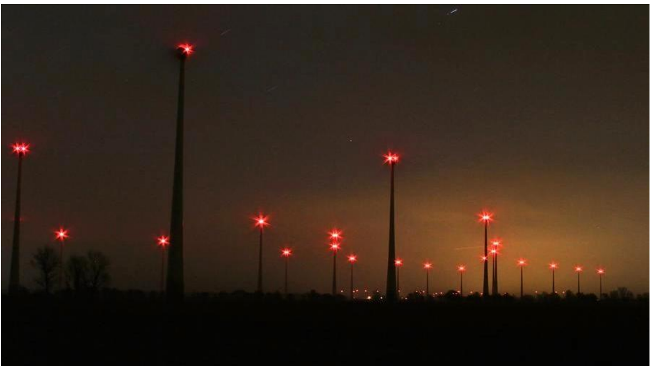
Figure 27: Example of aircraft warning lights fitted to the turbines as prescribed by the CAA 3
