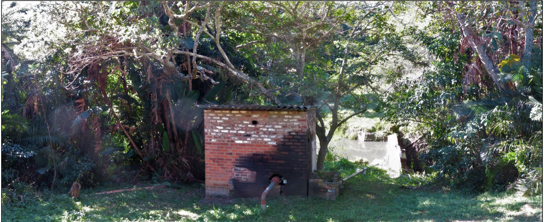
Plate 2: View of the existing abstraction works
