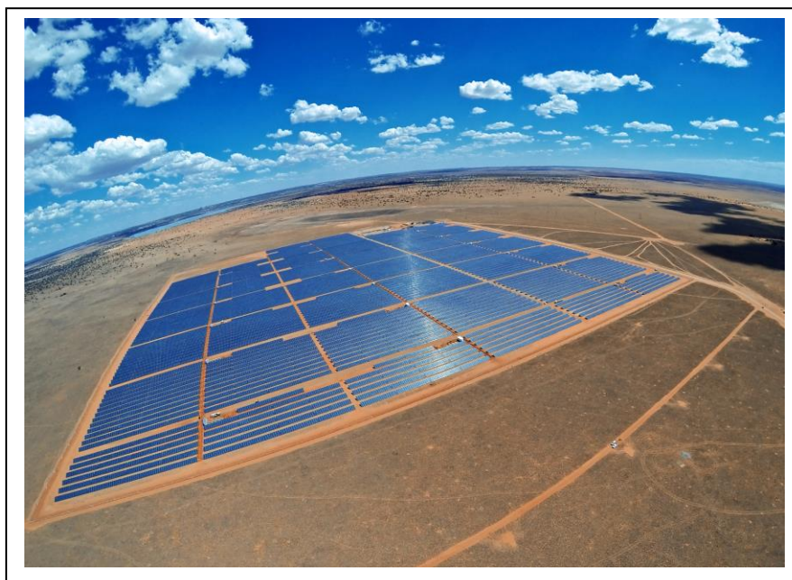
Figure 2.5: Photovoltaic panel array (with permission from Genesis Eco-Energy)
