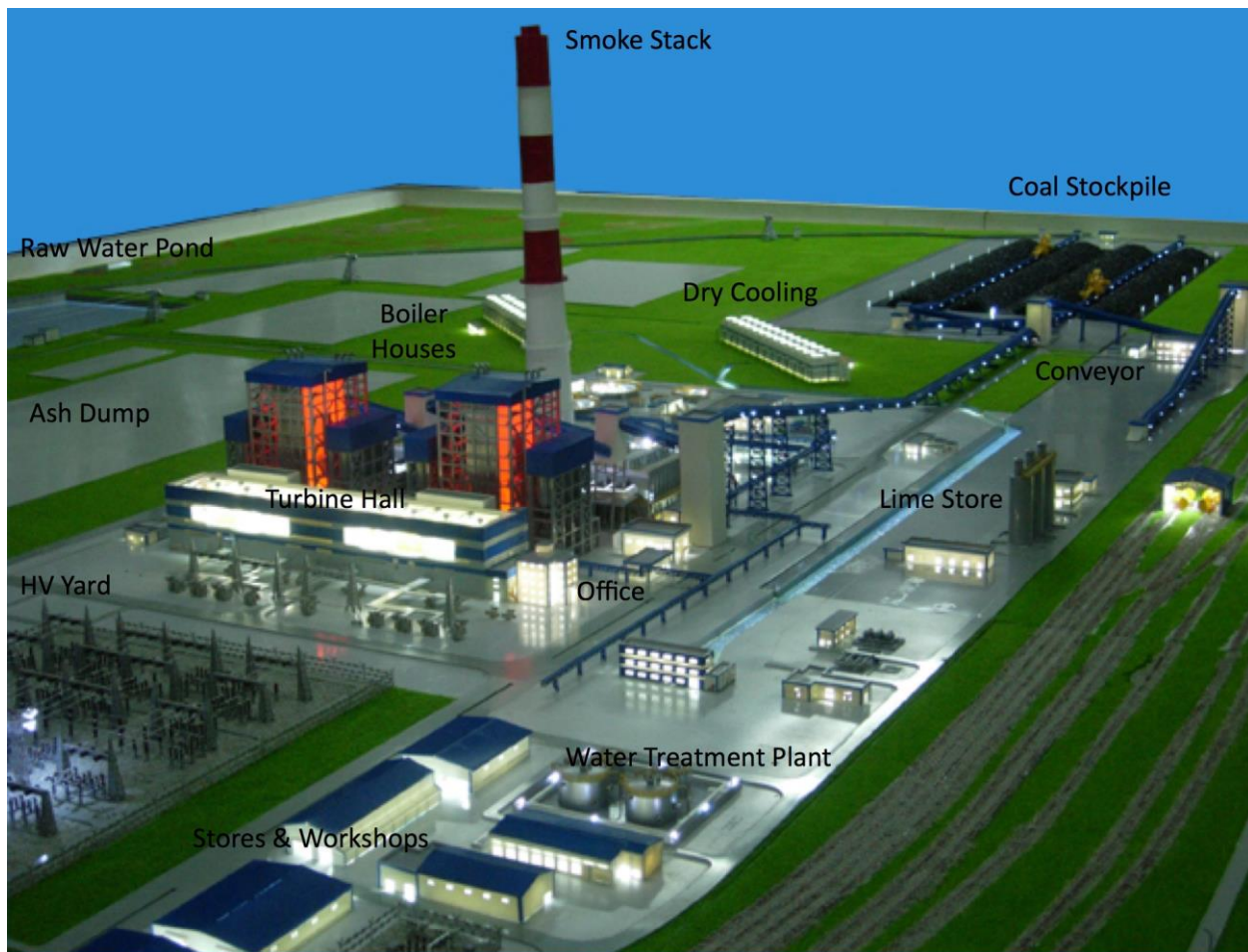
Figure 2.3: Typical CFB coal-fired power project layout. 3
