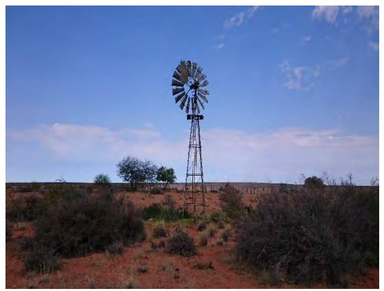
BH4 - wind pump
