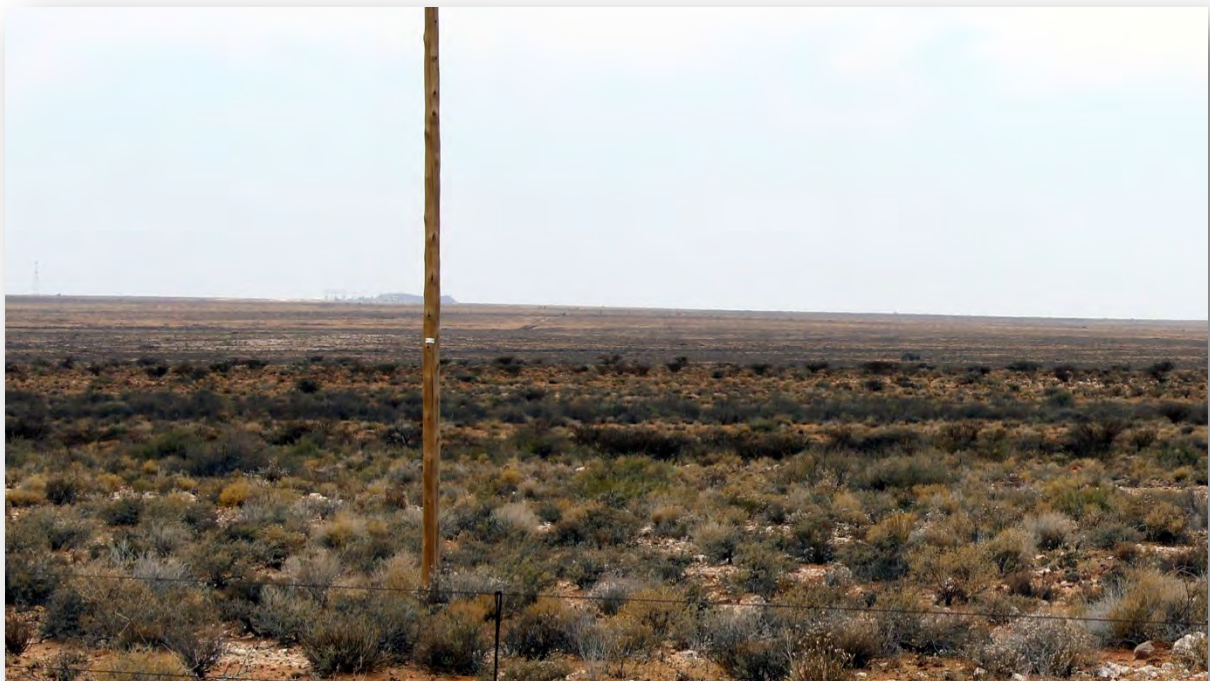
Figure 8.4: View from photo site SCA014 eastwards. The tower at Rugseer Siding is visible on the left and the new substation more towards the centre.
