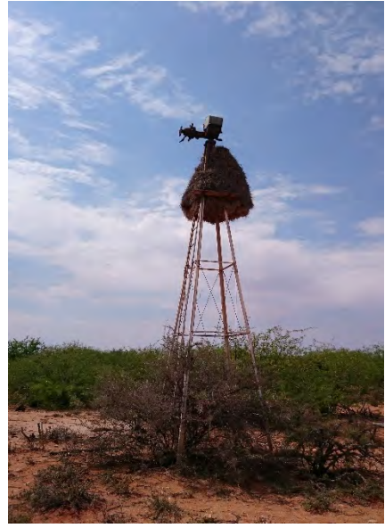
BH8 - wind pump
