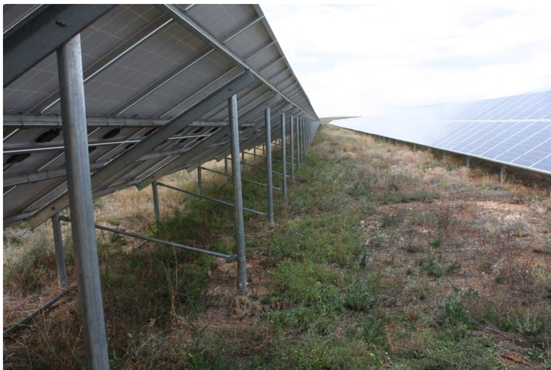
Figure 7.8: Image of solar arrays indicating the limited influence that such structures generally have on the flow of surface waters within a solar facility.
