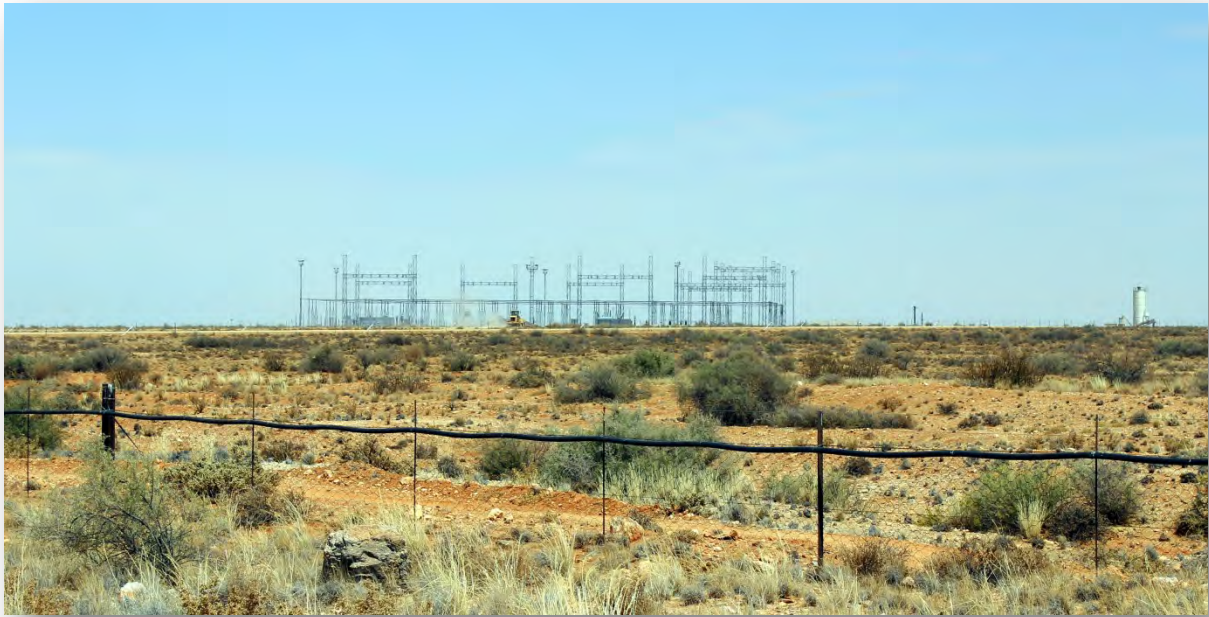
Figure 8.5: Nieuwehoop Substation currently under construction (Photo site SCA010)
