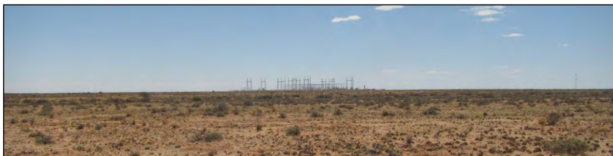
Figure 9.3: View towards the northeast (from the PV 1 site just north of the railway line) of the Nieuwehoop Substation currently under construction.
