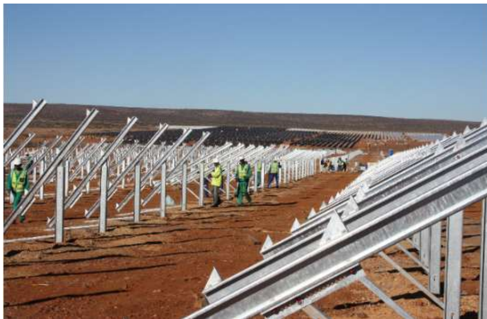
Figure 2.9: Frame, structural details (Lesedi Solar PV Project, Kimberly, South Africa. Source: Power Technology.com)
