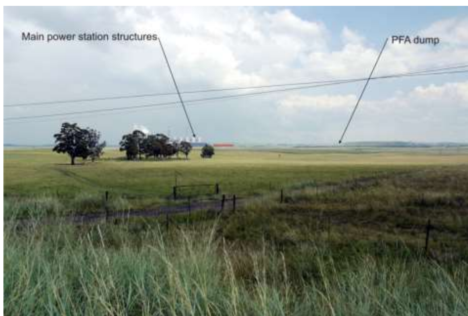
Figure 6.10: VP 4. View from local road to the east.
