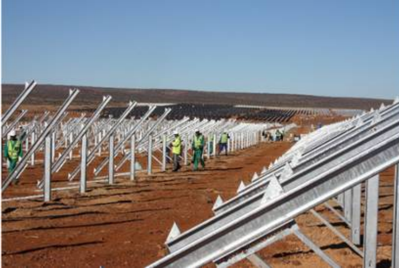
Figure 2.8: Frame, structural details (Lesedi Solar PV Project, Kimberly, South Africa. Source: Power Technology.com).
