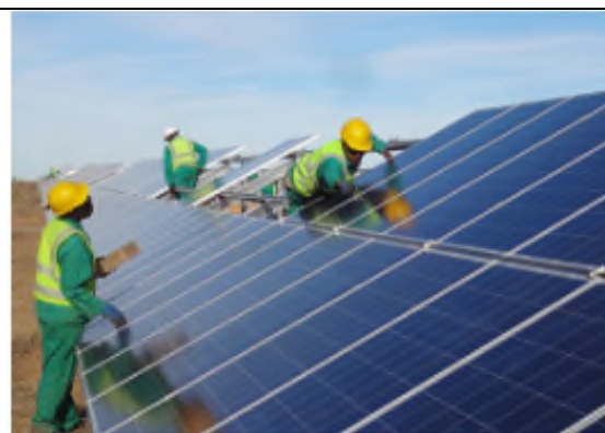
Figure 2.4 Picture of the installation of a typical PV array (75 MW plant in Kalkbutt South-Africa Source: PennEnergy)
