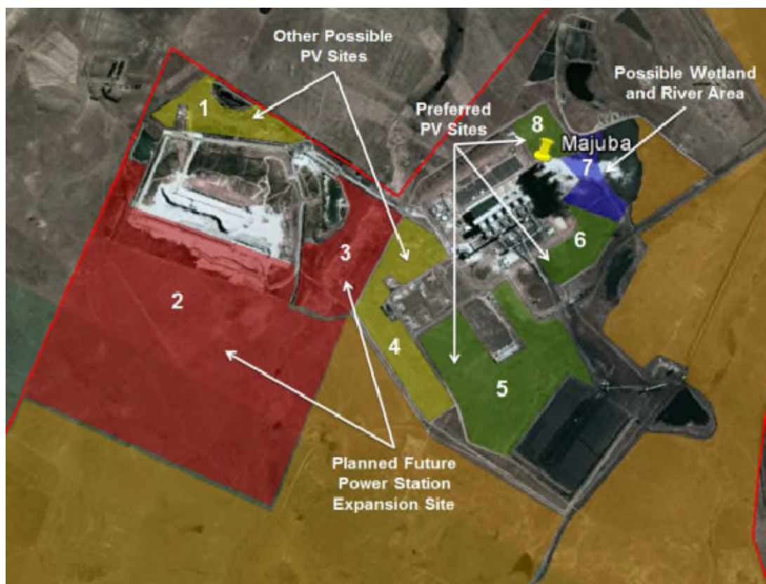
Figure 2.1: Aerial view of zoomed in area of Majuba power station with coloured areas as possible identified PV sites.
