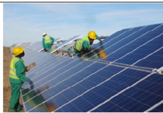
Figure 2.3: Picture of the installation of a typical PV array (75 MW plant in Kalkbutt South-Africa Source: PennEnergy)
