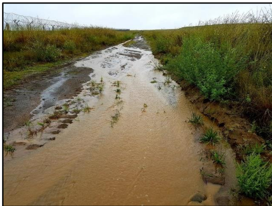
a) Stormwater runoff along service road.
